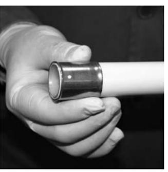
Insert the stainless steel cap into the tube, in the position that the inspection holes are located at the end of the tube.
