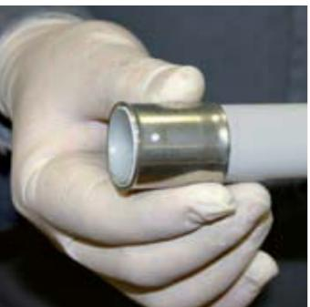
Insert the stainless steel cap into the tube, in the position that the inspection holes are located at the end of the tube.
